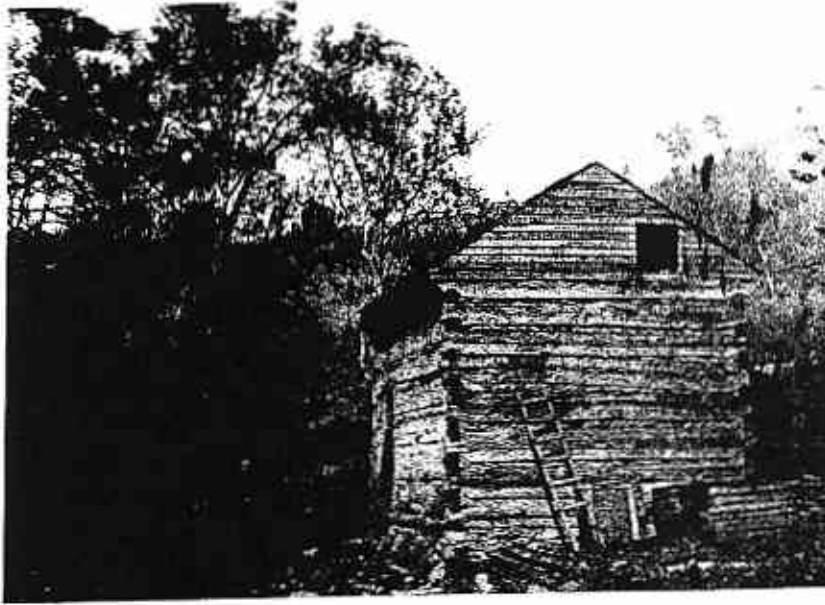
First log cabin built in Cincinnati, 1788, on Front Street, a fair east of what is now Main. "The hardy pioneers burnt their bridges behind them by breaking up the boats in which they came, to help construct their houses." Credit: Gots.
